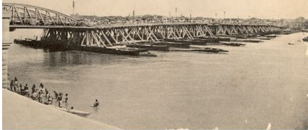
27. Hoohly Bridge, Howrah End, Calcutta
